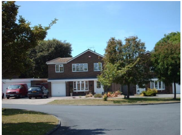
Sympathetic garage extension
